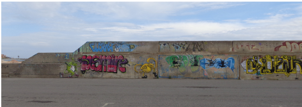
Figure 10. Maintenance of seawalls, Almerimar (Almería), ES.
